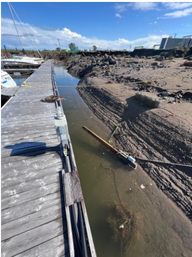
Note: The severely washed out areas destroyed approx. 6-8 feet of land all along 375ft of area
