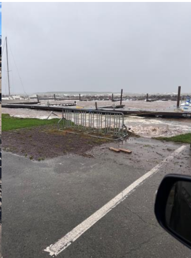
Note: The severely washed out areas destroyed approx. 6-8 feet of land all along 375ft of area
